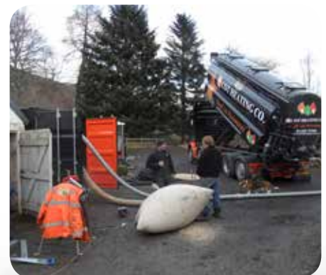
Adding pellets to the storage container, with the Basset colleague looking on.
